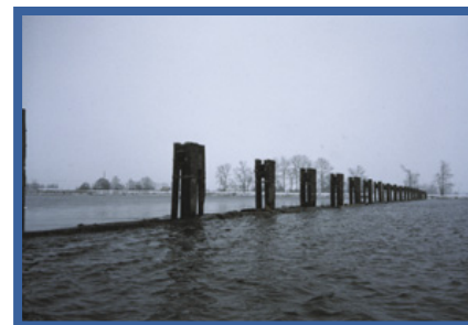
Floating breakwaters such as this one in the Fraser river can be designed to reduce the erosive energy of wakes.
