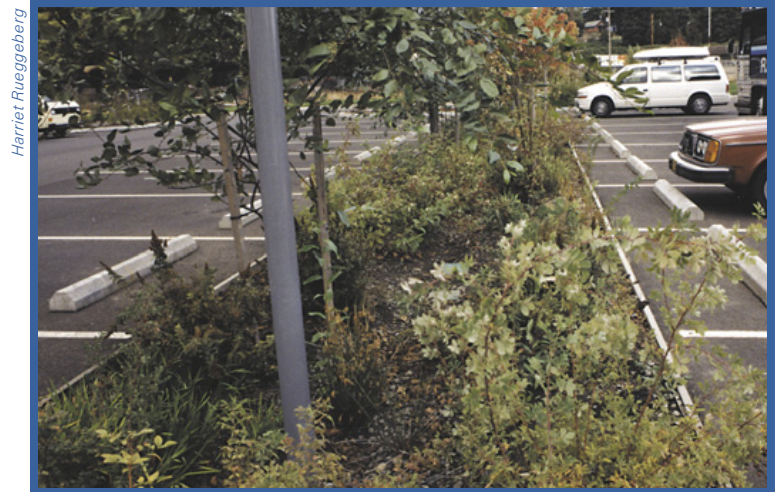
Surface runoff is captured in a marshy depression and dissipates slowly into the ground.
