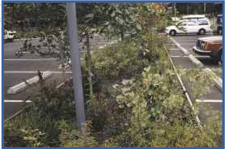
Surface runoff is captured in a marshy depression and dissipates slowly into the ground.
