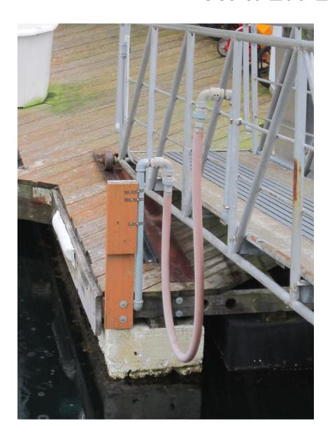
•ROTATING CONNECTIONS ON BOTH ENDS ALLOWS FOR A SHORTER LOOP THAT WILL STAY OUT OF THE WATER
