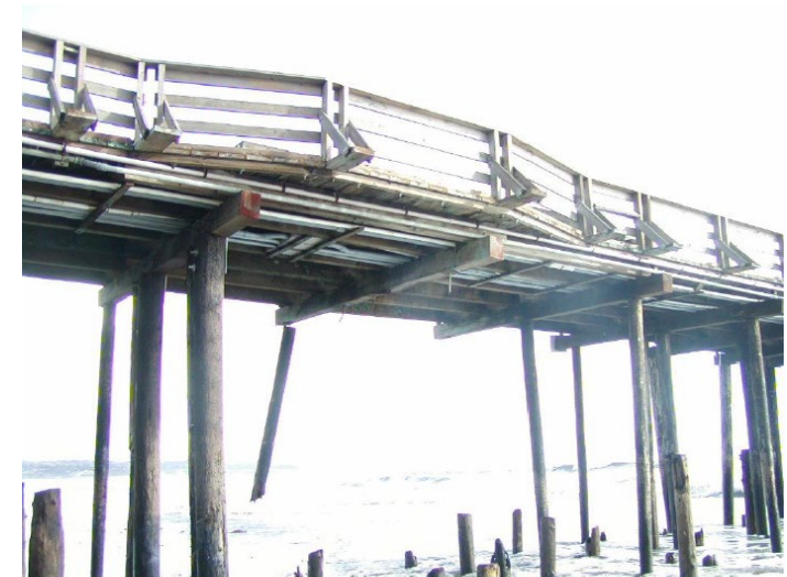
Photograph 10-All Piles Broken at Bent 12 (2002)
