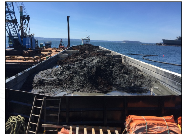
Flat-deck barge typically used to transport contaminated material to an upland transload facility
